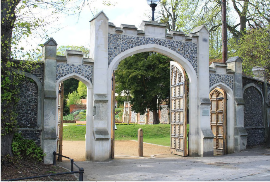
Stable Block Boundary Wall & Gate Piers from Highway
