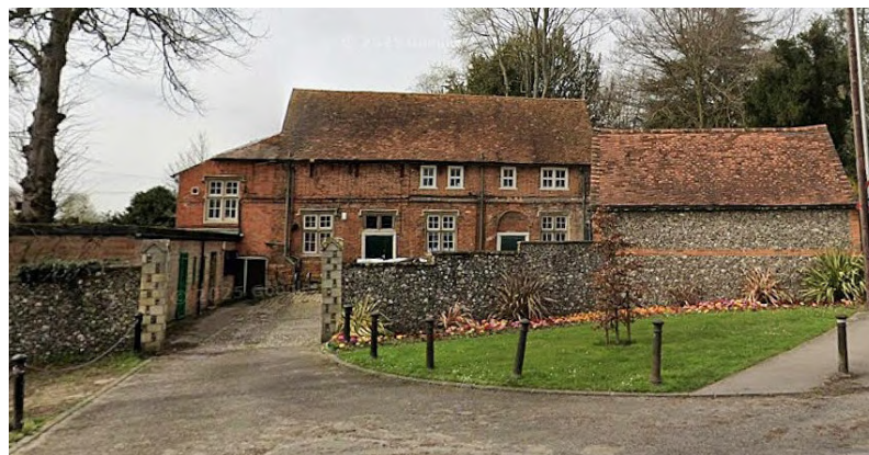
Stable Block Boundary Wall & Gate Piers from Highway
