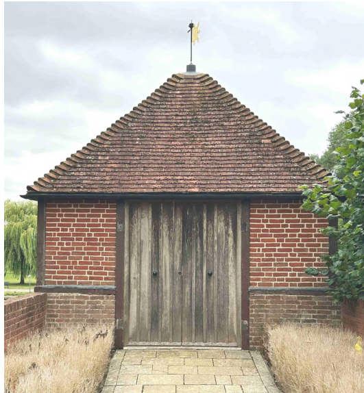
Gazebo External- North
