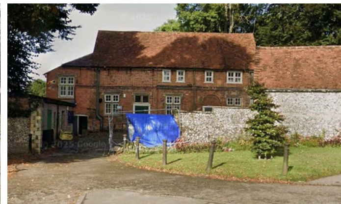
Stable Block Boundary Wall & Gate Piers Showing Damage from Highway
