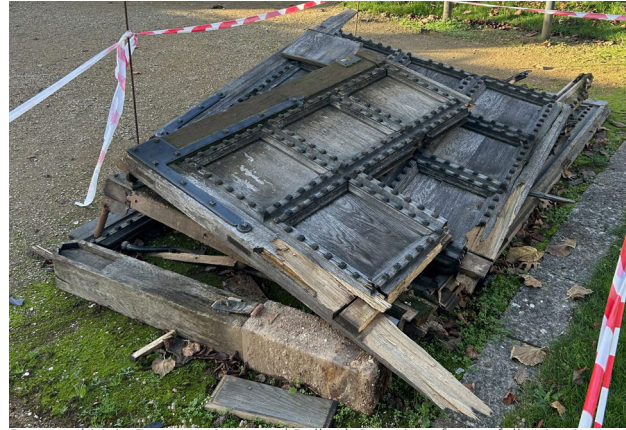
Damaged Main Entrance Gates and Bollard: Remains of gates following impact damage by car.
