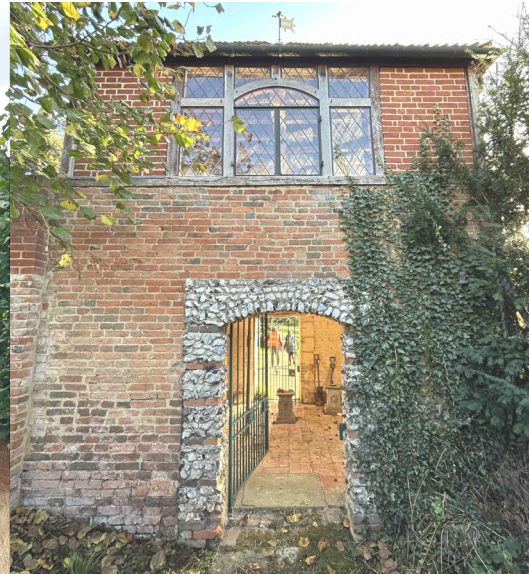
Gazebo External- West
