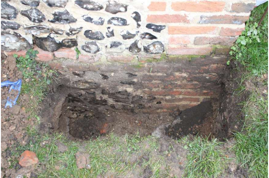
Fig. 4.21 Trial pit looking at south elevation
