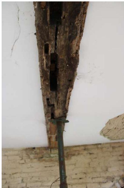
Fig. 4.32 Mortice holes and prop to main timber floor beam
