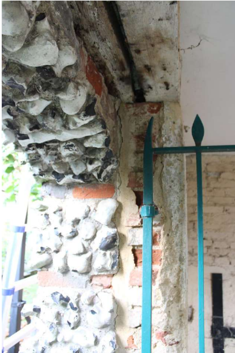
Fig. 4.37 Ground floor – west elevation at north side of gate opening.
