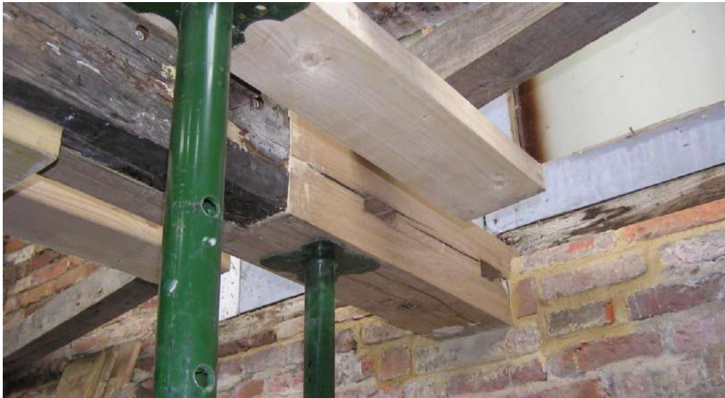
Fig. 5.1 First floor – repair work to north end of main beam in 2008
