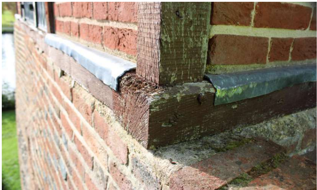
Fig. 4.3 North elevation – northeast corner post and plate
