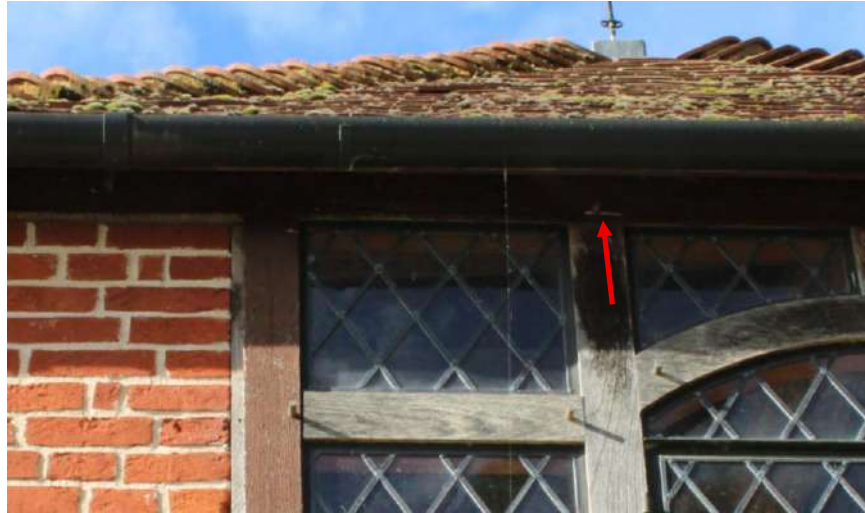
Fig. 4.11 East elevation – split above window post
