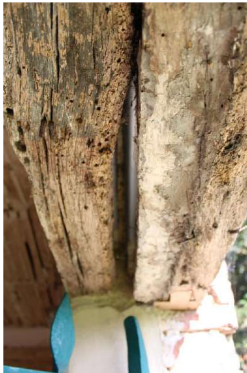
Fig. 4.8 East Elevation – lintels above gate
