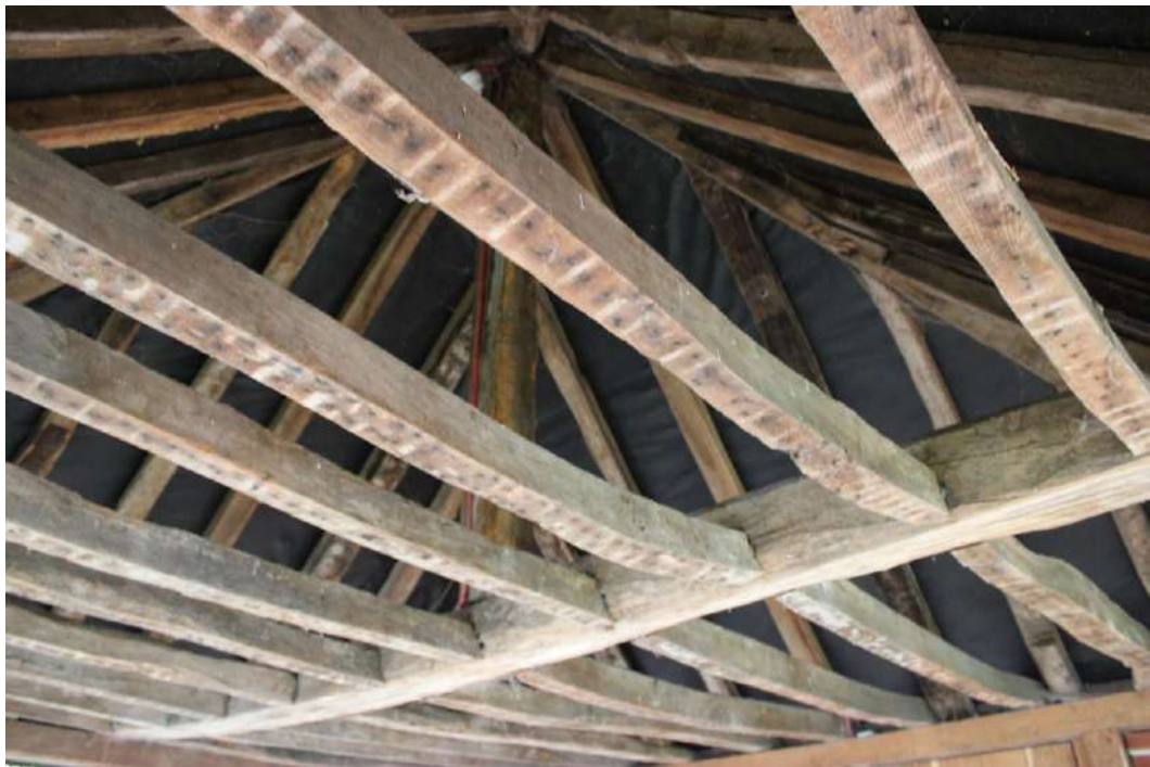
Fig. 4.38 General view of pyramid timber roof
