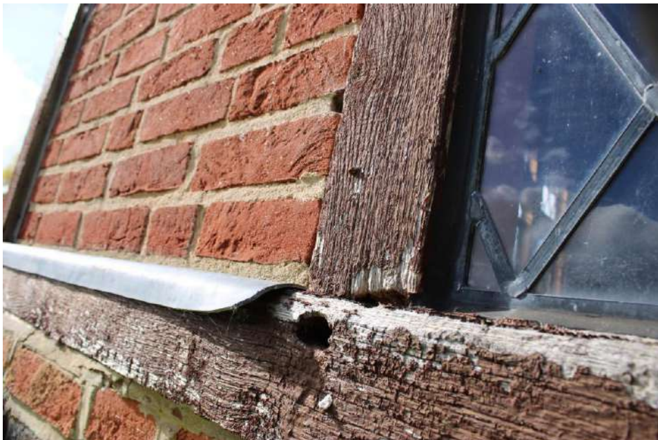
Fig. 4.10 East elevation – south window post
