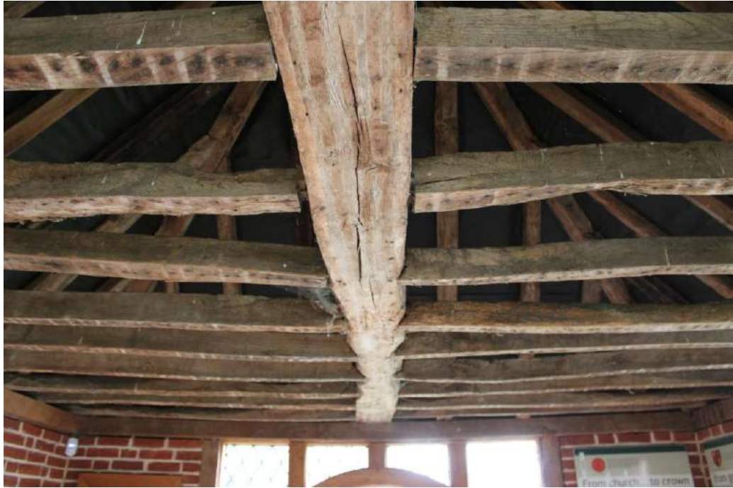
Fig. 4.46 First floor – central roof beam looking east (south side on the right – joints with ceiling joist do not suggest recent movement)
