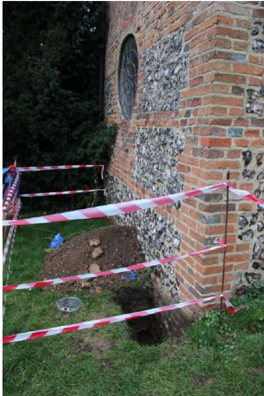
Fig. 4.19 Trial pit position
