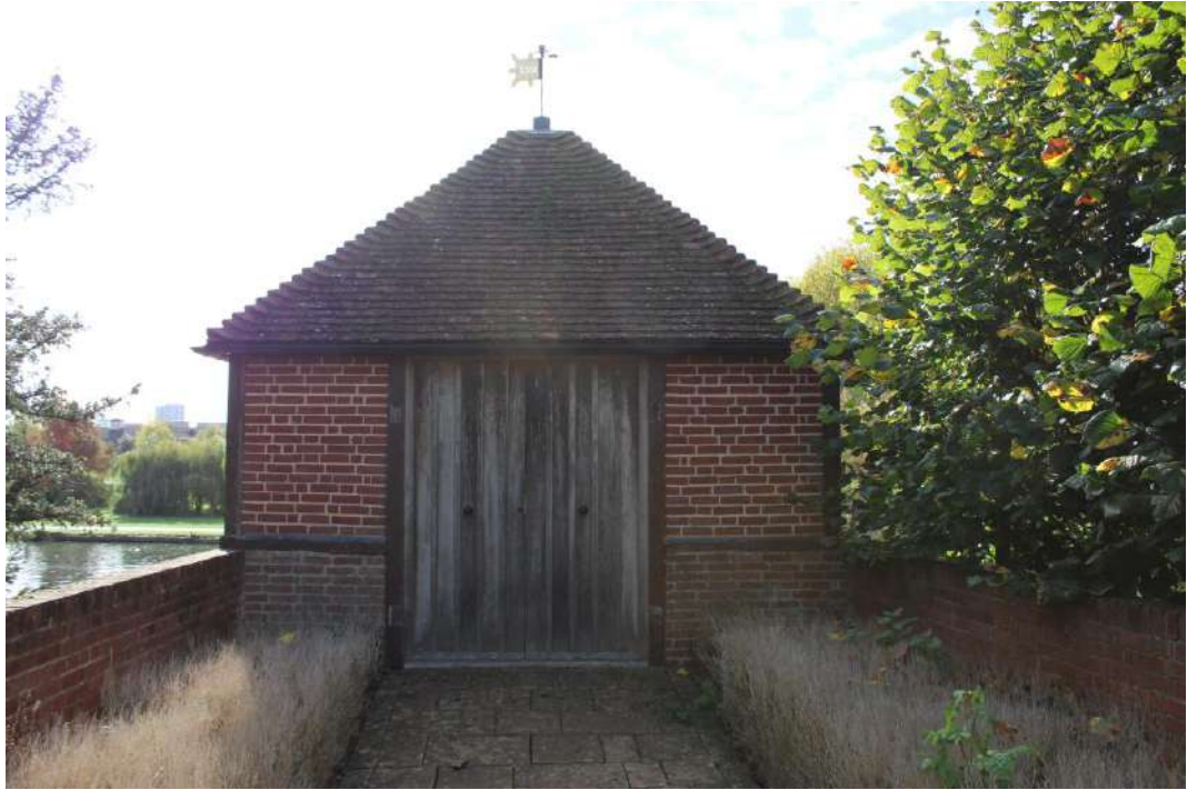
Fig. 3.2 Gazebo, North elevation (from causeway)
