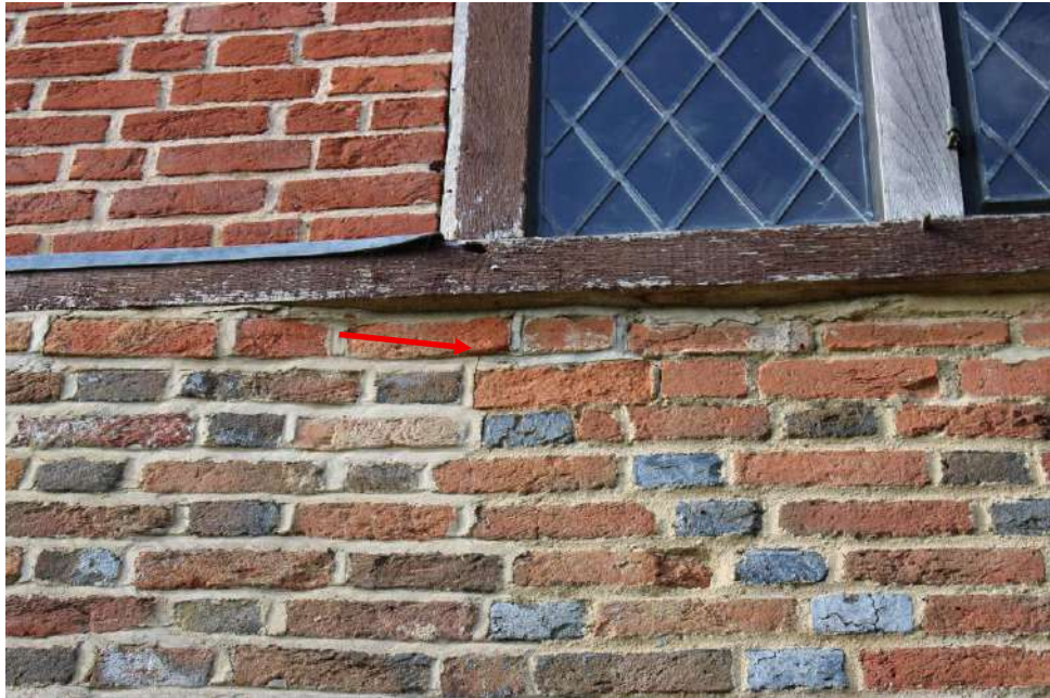
Fig. 4.9 East elevation – brickwork below south edge of window
