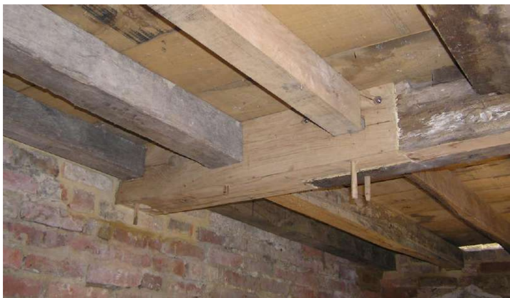
Fig. 5.2 First floor – repair work to north end of main beam in 2008
