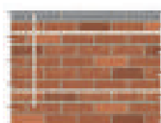
Securing parapet walls
