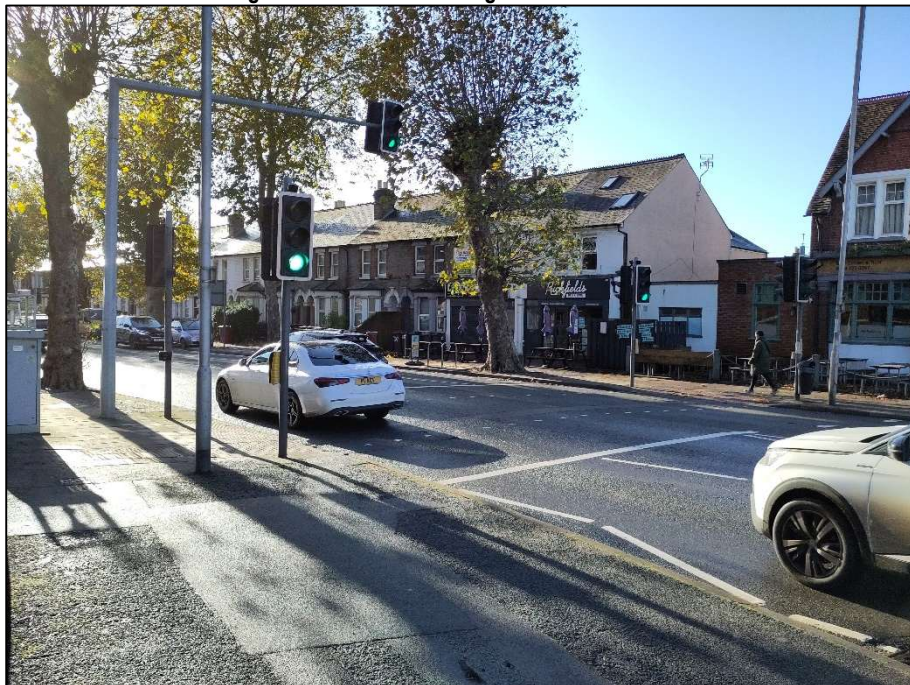
Figure 8.1: Toucan Crossing on Caversham Road
