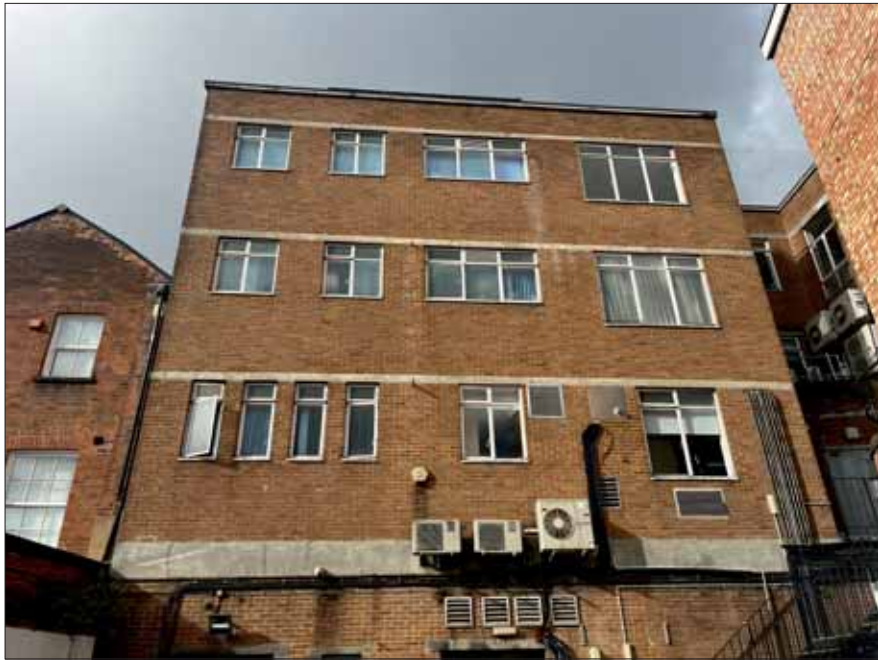
Photograph 2: Showing the rear of the building.
