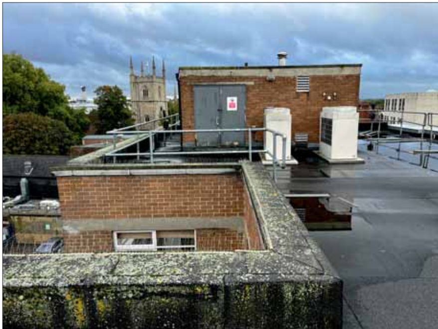
Photograph 3: Showing the flat roof and service unit.
