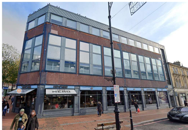
Existing western elevation (St Mary's Butts).
