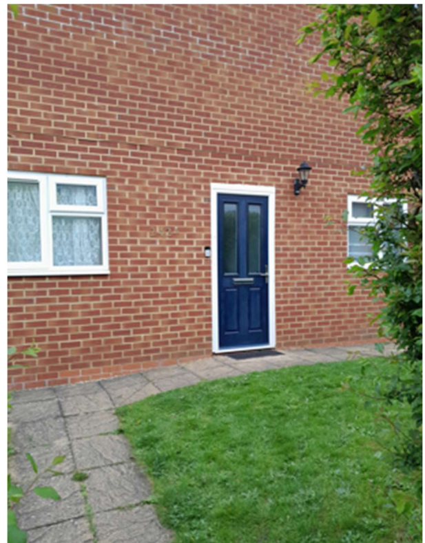
Existing front door in elevation facing Frogmore Way.
