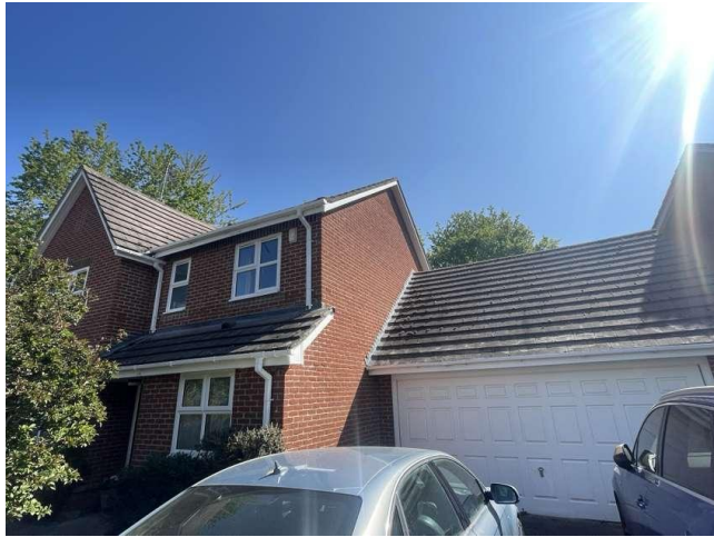
Photo 1: Southern and western elevations of B1
