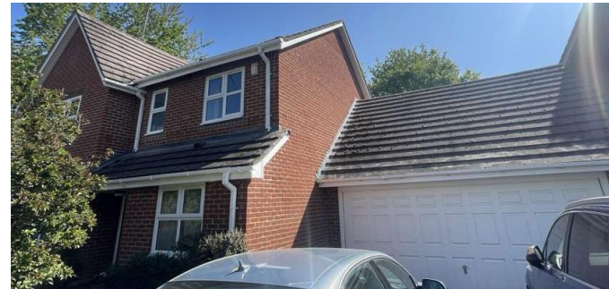
Southern and western elevations of B1
