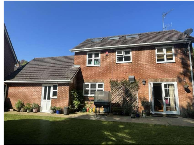
Photo 2: Eastern elevation of B1
