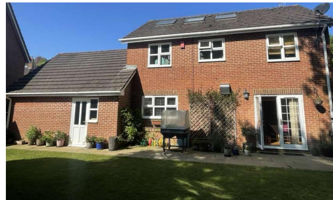
Eastern elevation of B1
