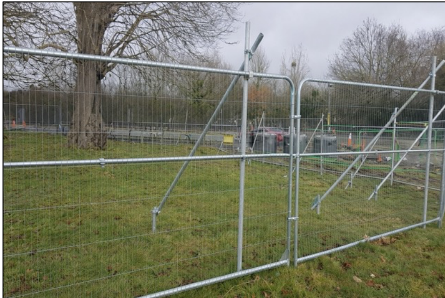
TPB 1 — Scaffold framework with weld mesh panels and back-stays
