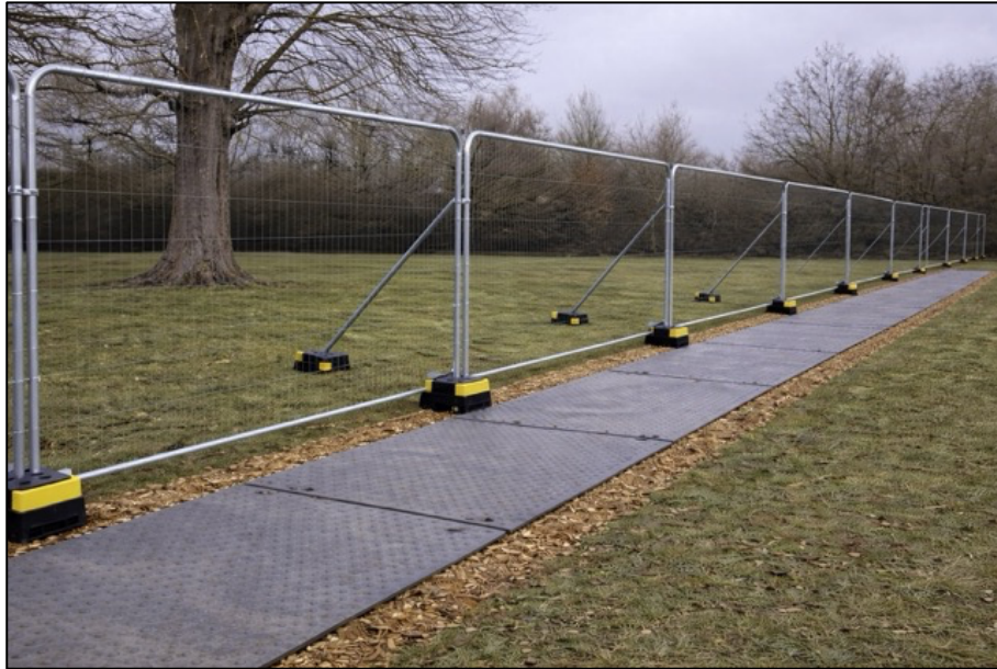
Ground protection example — woodchip and trackmats
