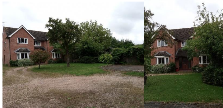
Existing front of the detached dwelling
