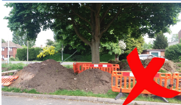
Unacceptable example of tree protection due to a lack of adequate fencing and poor site management. Note mounds of soil have been placed within the Root Protection Area.
