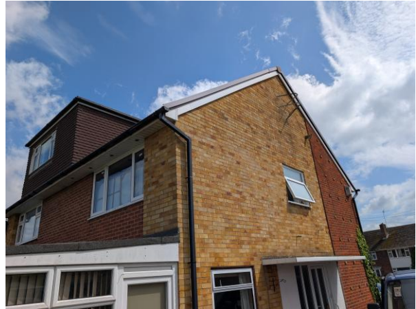
Photograph 2. The side elevation of the dwelling.
