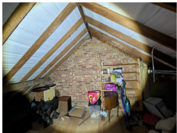
Photograph 6. Detail of the loft space of the dwelling.
