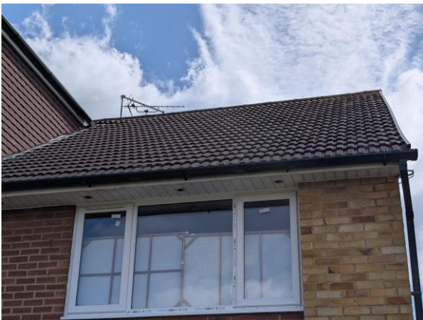
Photograph 3. Detail of the roof to the northern elevation of the dwelling.
