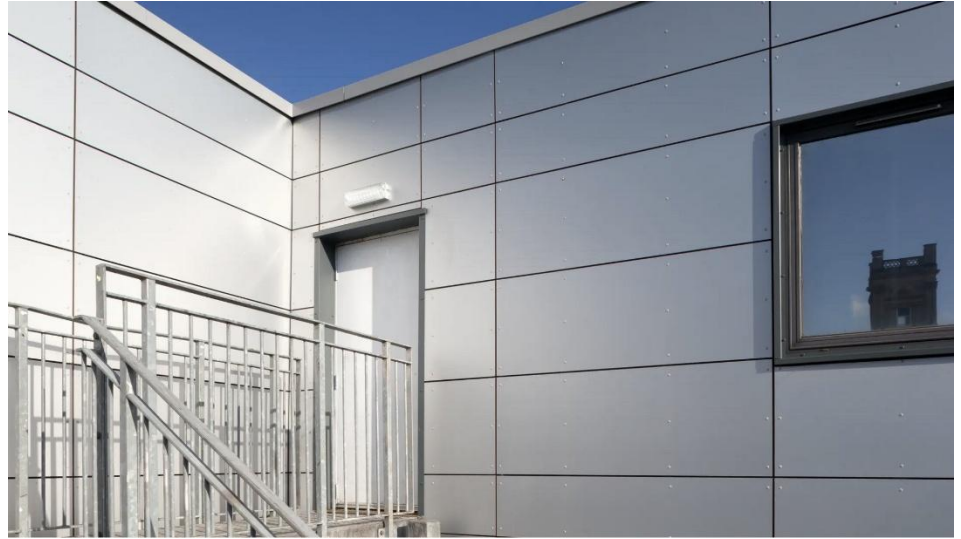
Above: Example of Rockpanel cladding completed
