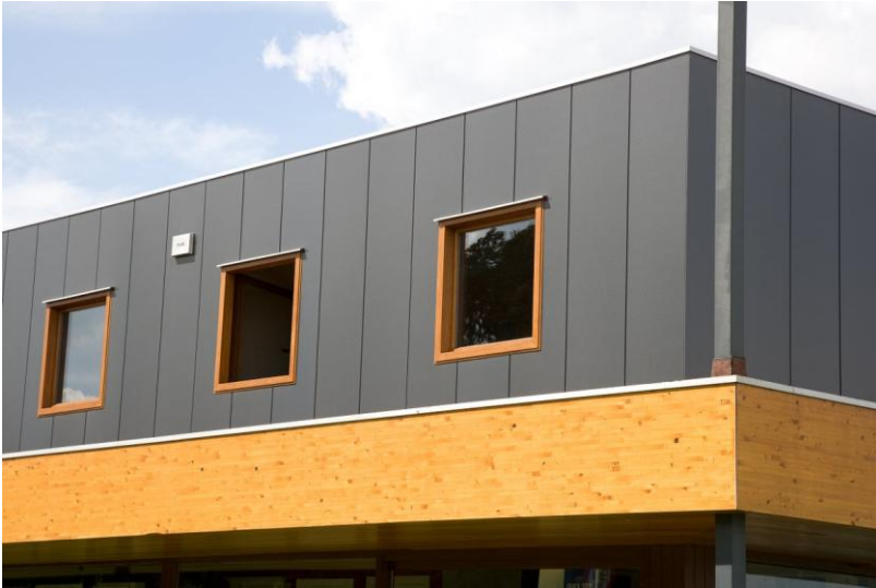
Above: Example of Rockpanel cladding during installation process
