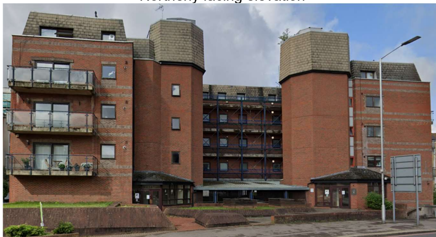
Easterly facing elevation
