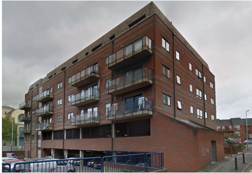
Westerly and southerly facing elevations
