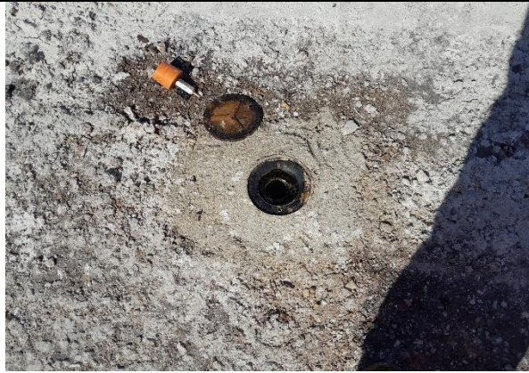
2. Flush headworks in place before GGS modifications.
