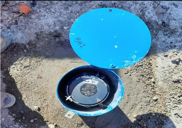
4. Instrument installed within headworks.
