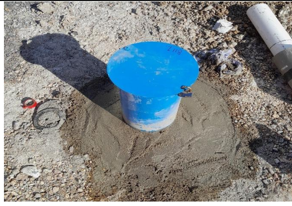
5. Headworks secured.
