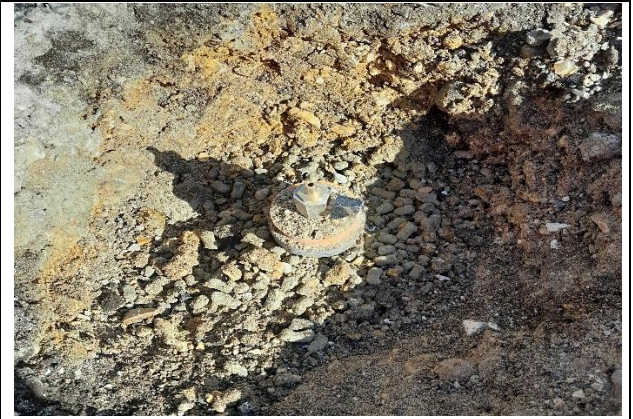
3. Standpipe before GGS modifications.
