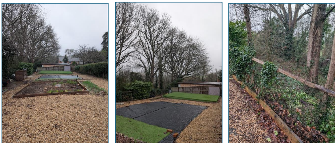
Proposed site showing foundations in situ, covered with green tarpaulin. Woodland to North (left of picture) approximately 1m below level of proposed site.
