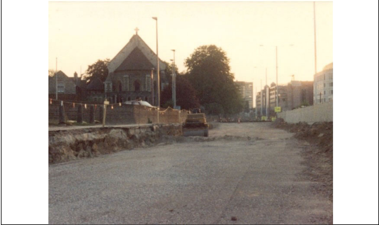
Figure 5 Excavation of the IDR. Image Gareth Thomas 1989. Courtesy Reading Borough Libraries. The (now demolished) Metal Box building and Apex Plaza are on the right, St James's Church and Forbury Gardens on the left.
