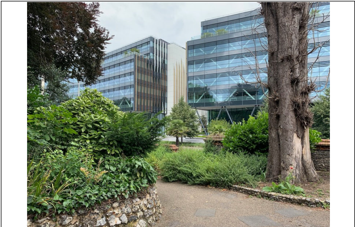
Figure 2 1 & 2 Forbury Place from the northern edge of the Forbury Gardens
