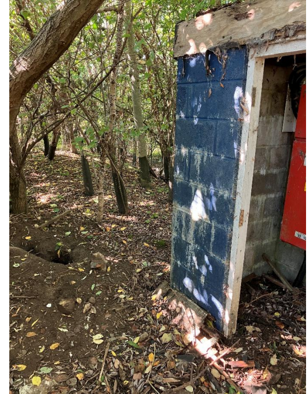
Plate 3: Badger holes by Building 1 in woodland
