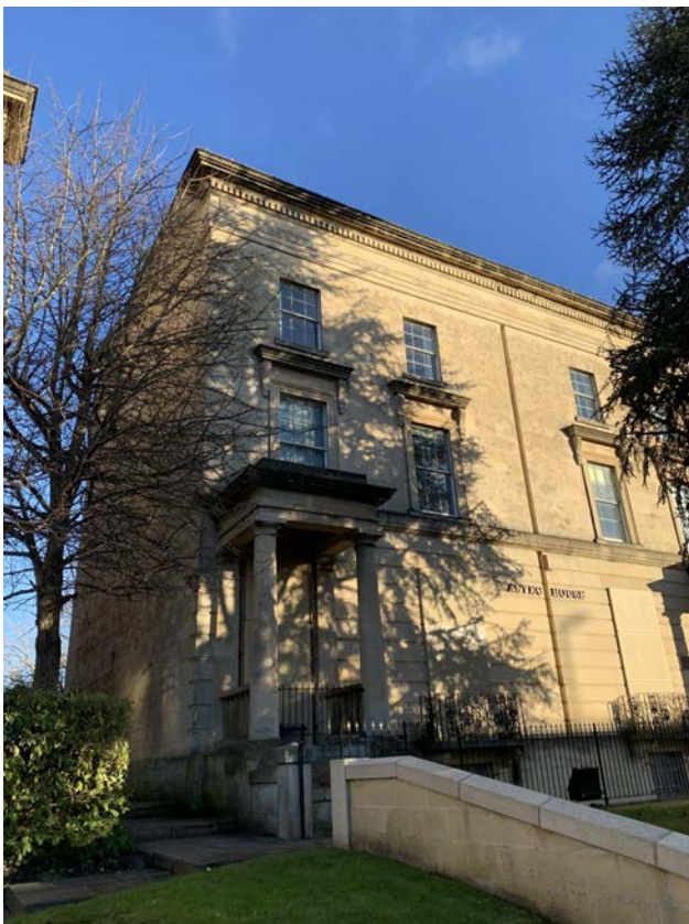
Photograph One - The front to the three storey building on-site, Aztec House.
