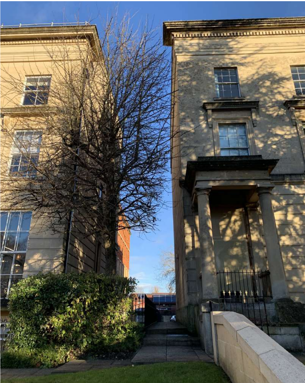
1 Front elevation with lefthand side stone porch, now redundant as an entrance.
