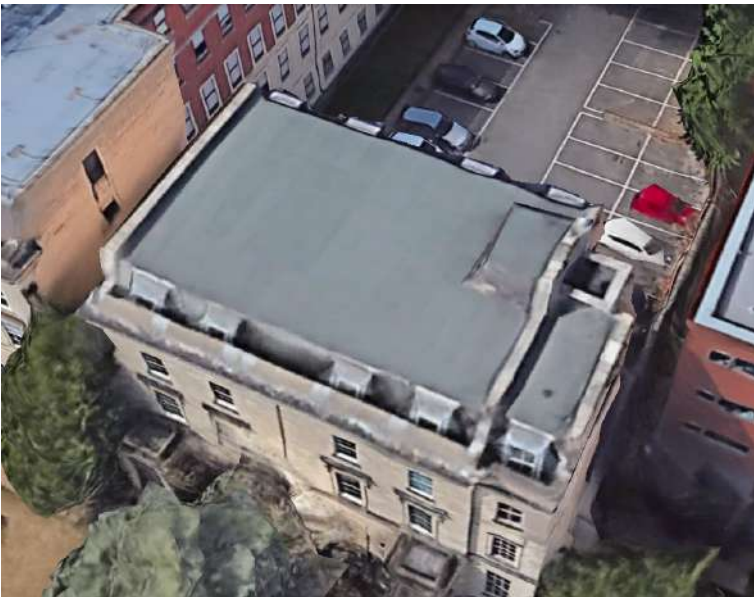
4 Google Earth view of the flat roof. The extension to the righthand side can be seen along with alterations for the lift shaft.
