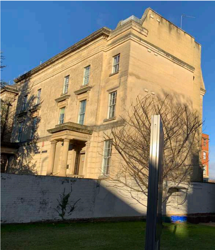
1 The flank elevation is more severe than the front elevation. The righthand side appears to be an extension to the original building.
