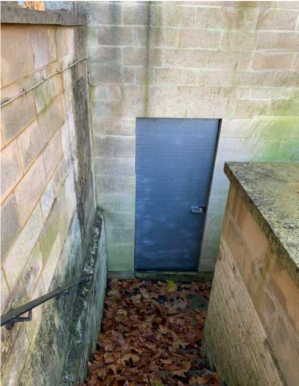
4 Stair to lower ground entrance to the plant room
