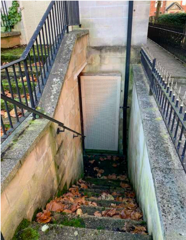
5 Stair to lower ground entrance at the rear frontage
