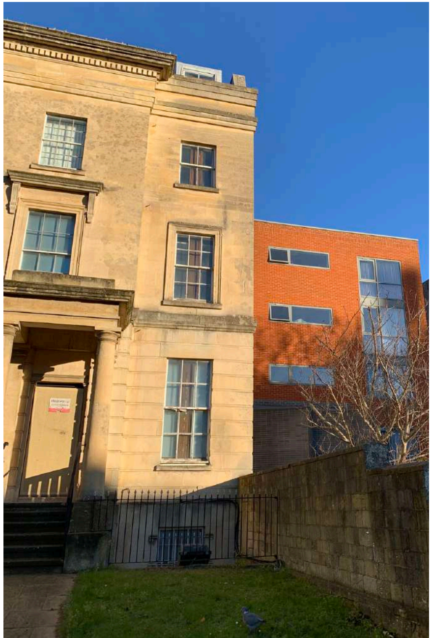
2 Front elevation with righthand side stone porch and main entrance. The righthand side is set back and simpler in detail from the main frontage.
