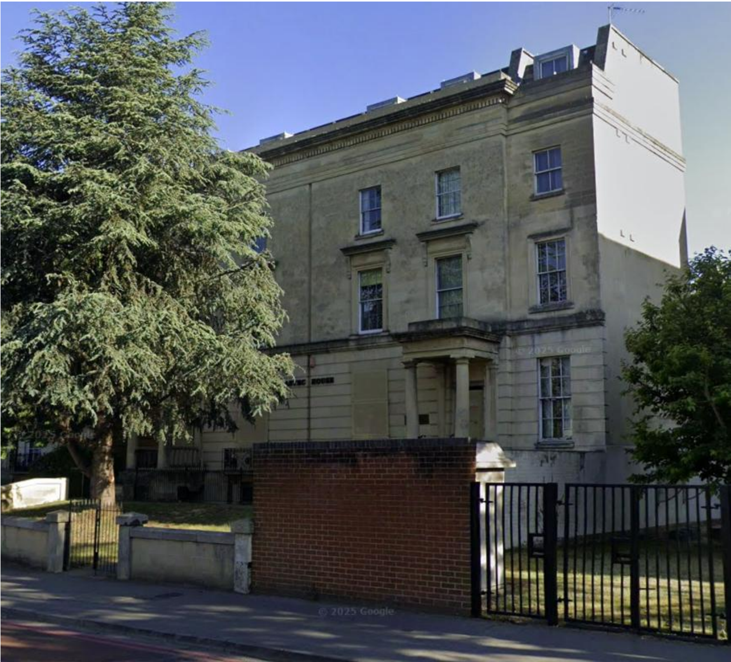
Figure 2. Existing stone façade of Astec House (source: Google Maps, accessed: December 2025).
