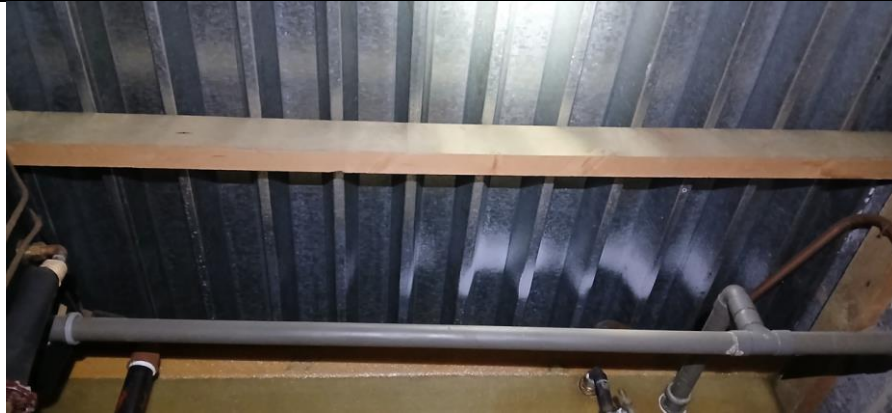
Figure 7 Internal ceiling of the boiler room within B1
