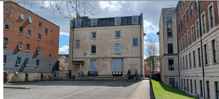
Figure 1 B1, northern elevation
