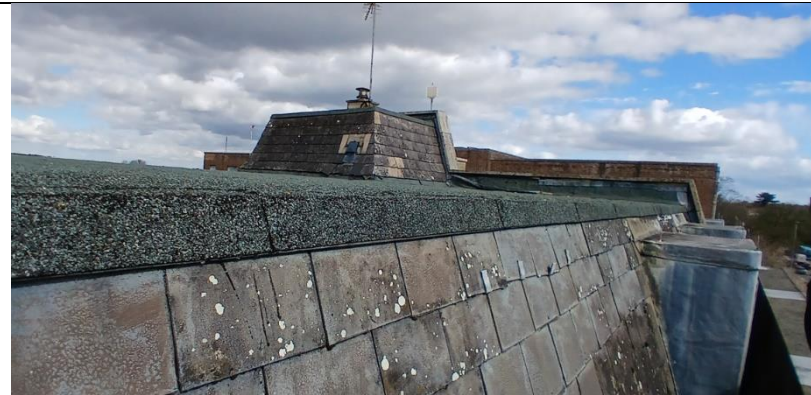
Figure 3 B1 roof, facing east
