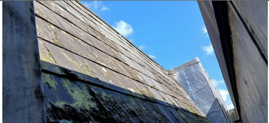
Figure 10 Angled slate tiles at the south of B1, facing east
