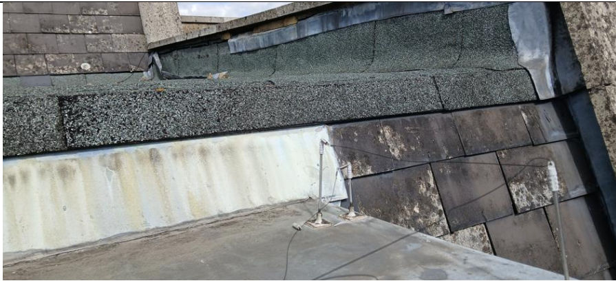
Figure 11 Well-sealed lead flashing at the south of B1
