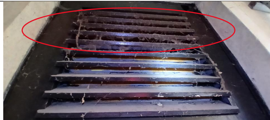
Figure 14 Airwave door leading to C02, with boarded area at bottom (Open access circled)
