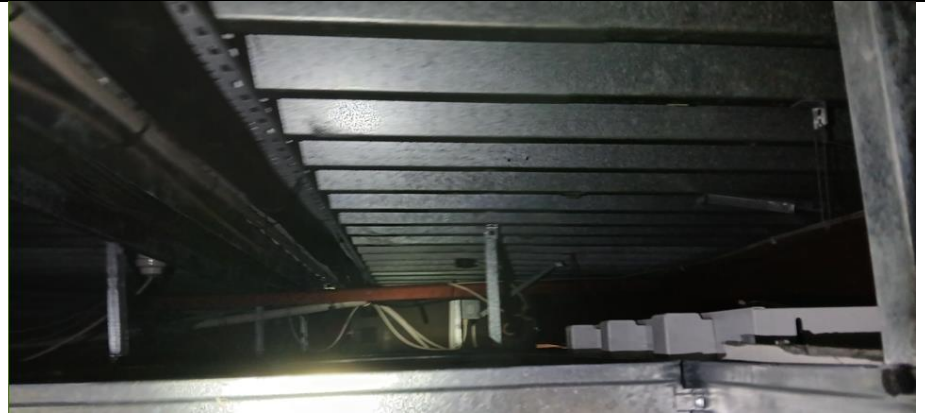
Figure 8 Space between dropped ceiling at the top floor in B1
