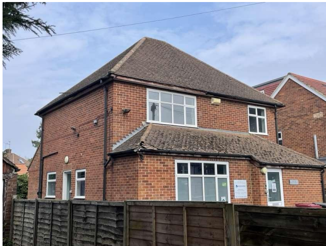
Photo 3: The southern and western elevations of B1
