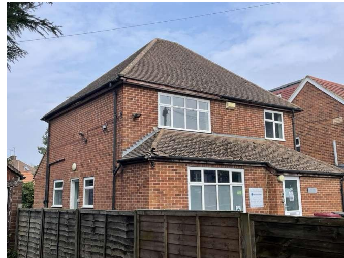
Southern and western elevations of B1
