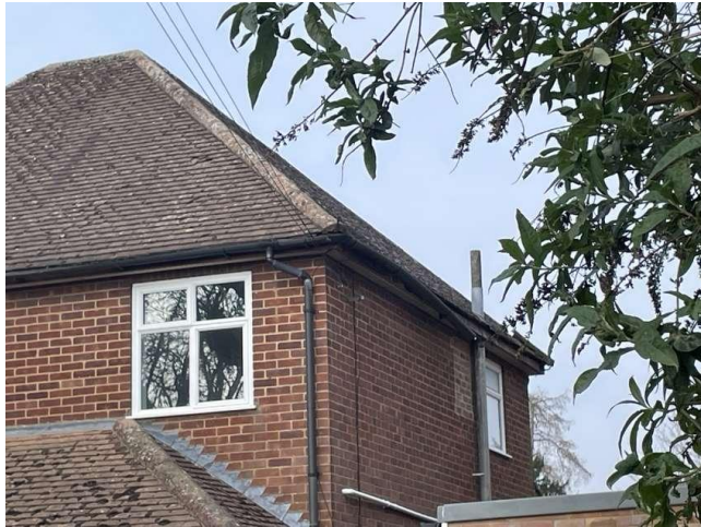
Photo 5: The eastern elevation of B1
