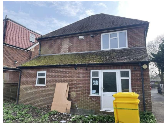
Northern elevation of B1
