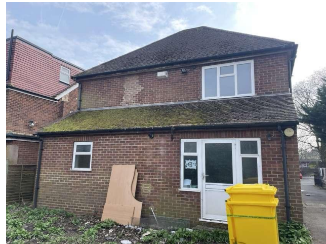
Photo 4: The northern elevation of B1
