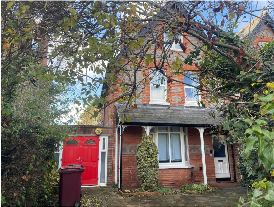
View of the application site and subject building at 8 Glebe Road
