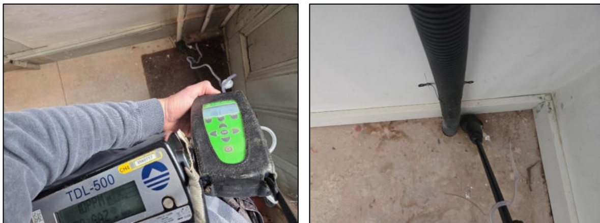
Figure 1 Selected GGS site photographs taken during the detailed gas sweep survey, including survey measurements targeting service entry points on the ground floor.
