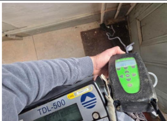
Measurement at service entry
