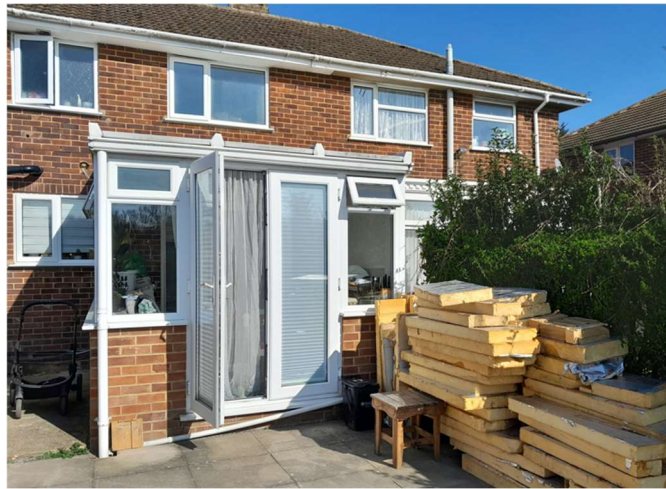
Looking north towards rear elevation
