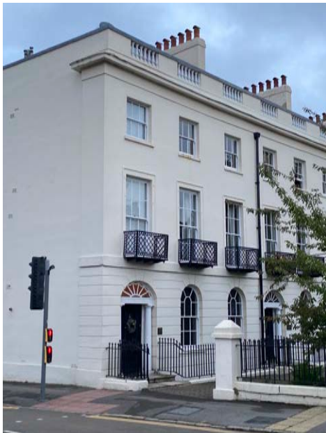
Fig.1: Photograph of western end of Albion Terrace viewed from corner of London Road and Sidmouth Street (apartment 7 located on second floor).
