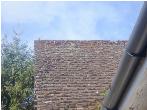
Photograph 11. Intact ridge mortar (south elevation).
