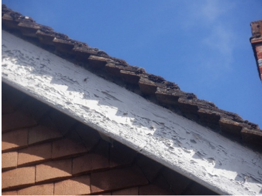
Photograph 13. Intact verge mortar and timber fascia (front elevation).
