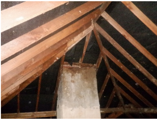
Photograph 19. Roof void with mostly intact bitumen roof felting (roof void).
