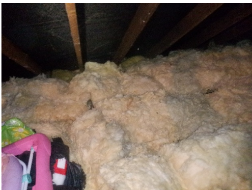
Photograph 23. Fibreglass between the joists and filling most of the eaves (roof void).
