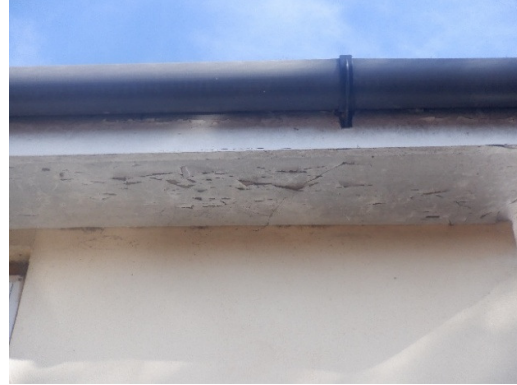
Photograph 14. Intact timber fascia to rendered brickwork of bungalow (front elevation).
