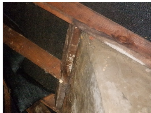
Photograph 24. Rendered chimney tightly fitted to timber rafters (roof void).
