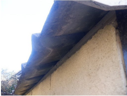
Photograph 17. Corrugated roof tight to rendered brickwork of outbuilding (western elevation).
