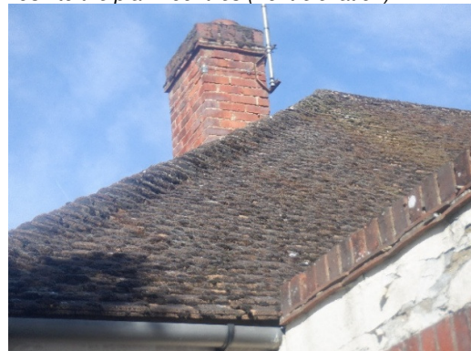
Photograph 12. Intact hip mortar (south-eastern elevation).
