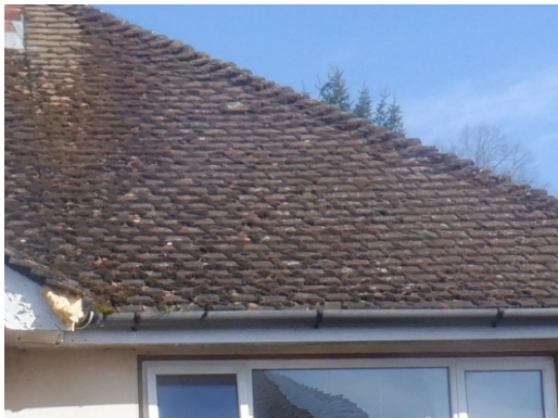
Photograph 9. Intact plain roof tiles (front elevation).
