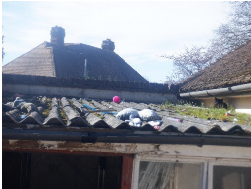
Photograph 16. Corrugated metal roof tight to brickwork and timber bargeboards of garage (rear elevation).
