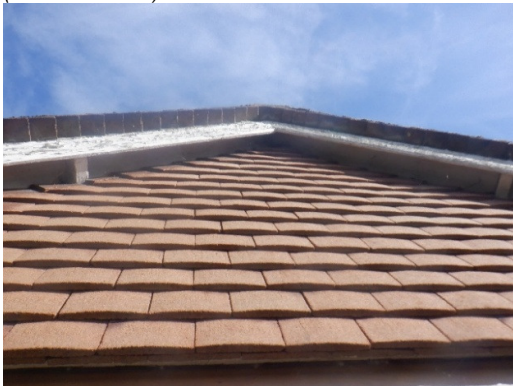
Photograph 15. Flat hanging tiled on gable end (front elevation).
