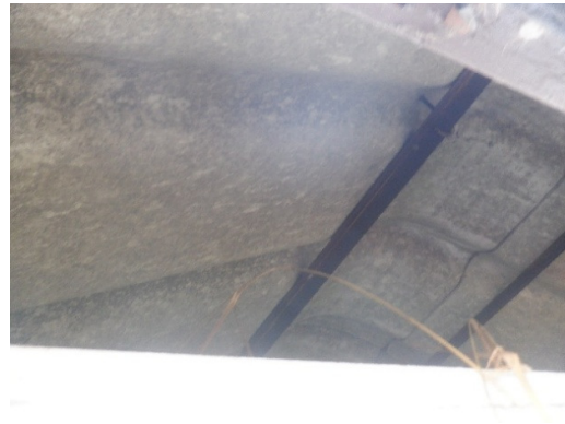
Photograph 28. Open to the underside of the corrugated asbestos sheeting (internal view of outbuilding).
