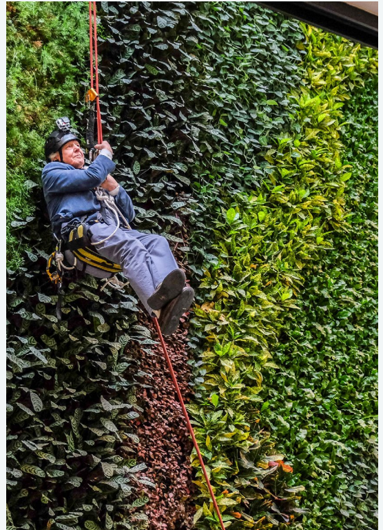
David Attenborough Building, installed in 2016
