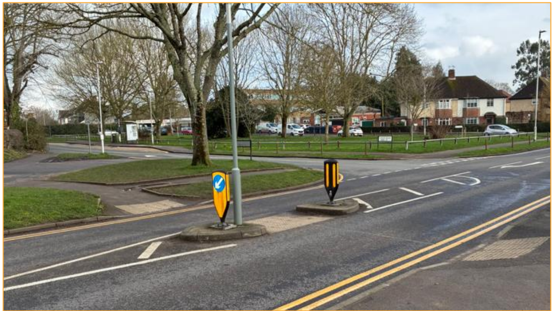
Figure 3 - Uncontrolled Crossing, Evesham Road / Grove Road
