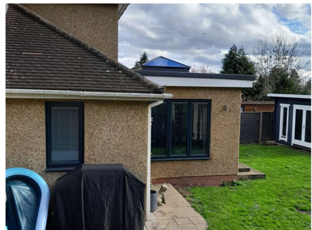
Existing side, north-westerly facing elevation
