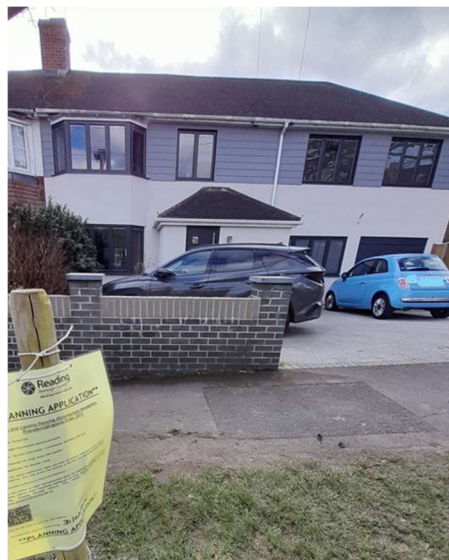
Existing front, north-easterly elevation
