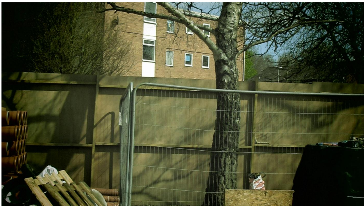
PHOTOGRAPH NO. 3 – Protective barriers around T3 – Silver birch (TPO No. 1 – 20/16)
