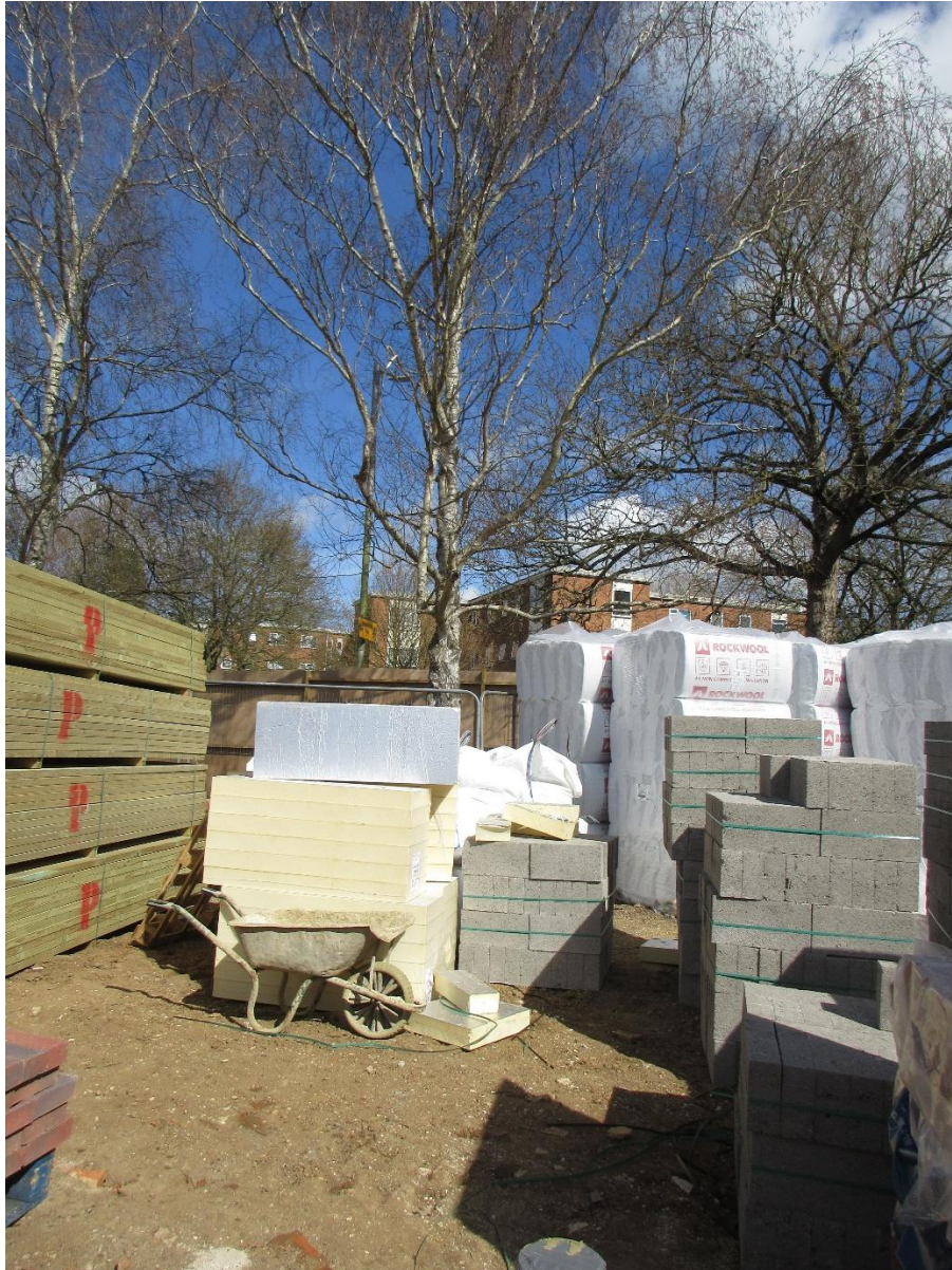
PHOTOGRAPH NO. 1 – Materials stored west and south of the trees
