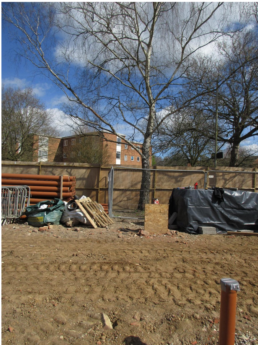
PHOTOGRAPH NO. 4 – Protective barriers around T3 – Silver birch (TPO No. 1 – 20/16) showing the lightweight plastic drainage goods to the left (northern) end
