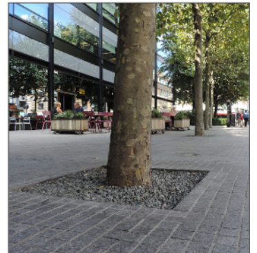
Paving recessed tree grille
