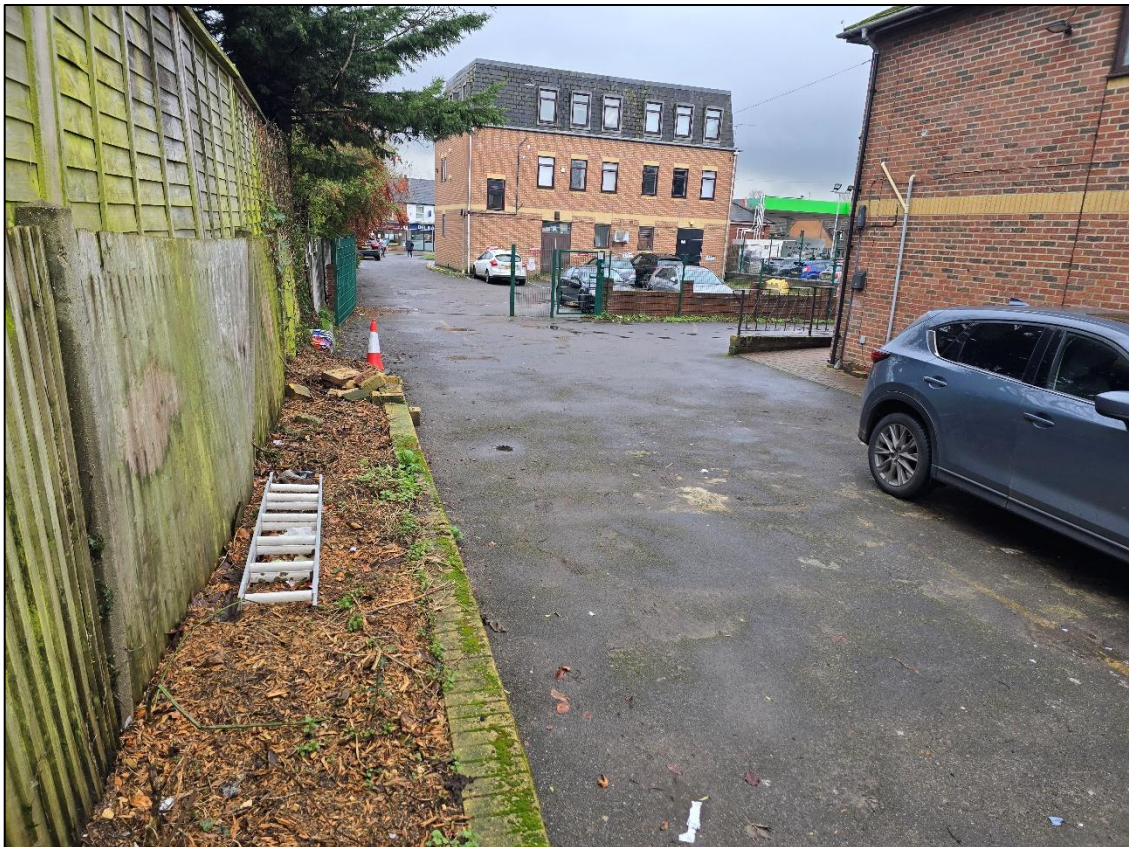
Photo 5. Low-level soft landscaped bed along northeast boundary to be protected with temporary ground protection
