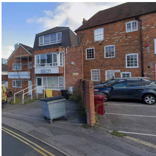
2. Existing refuse collection on Crossland Road
