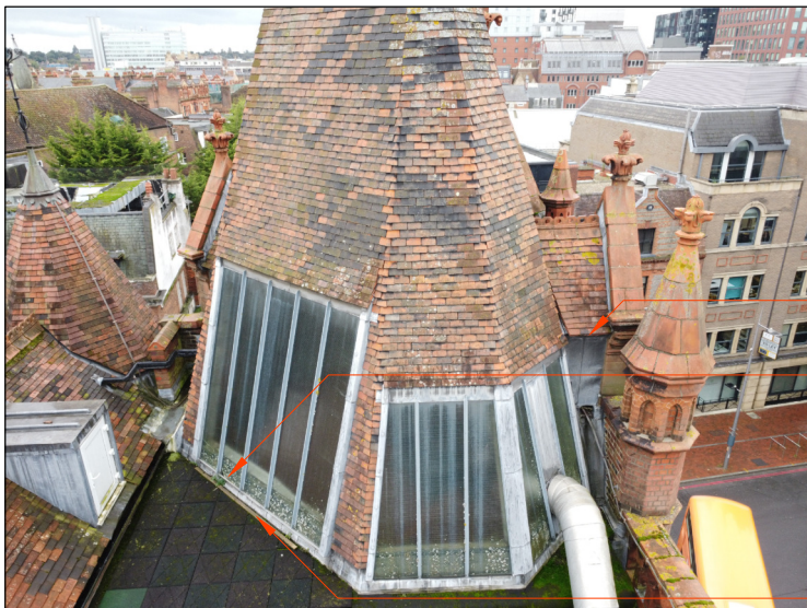
07 ROOF SLOPES AND PATENT GLAZING RF10 NTS - Date Taken: 09/10/24
