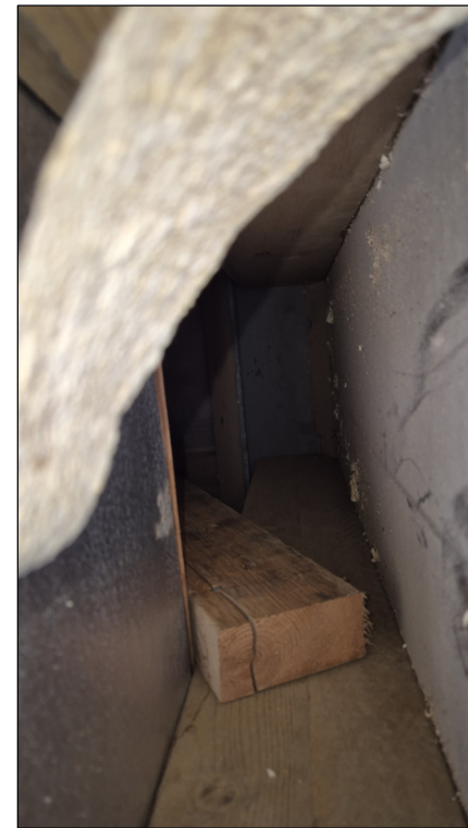
06 VOID BELOW VALLEY GUTTER NTS
