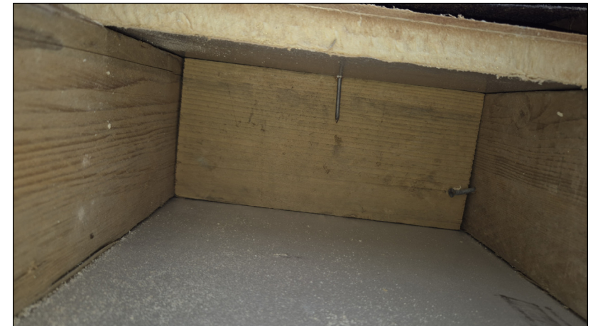
07 EXISTING TIMBER NOGGINS BETWEEN JOISTS NTS
