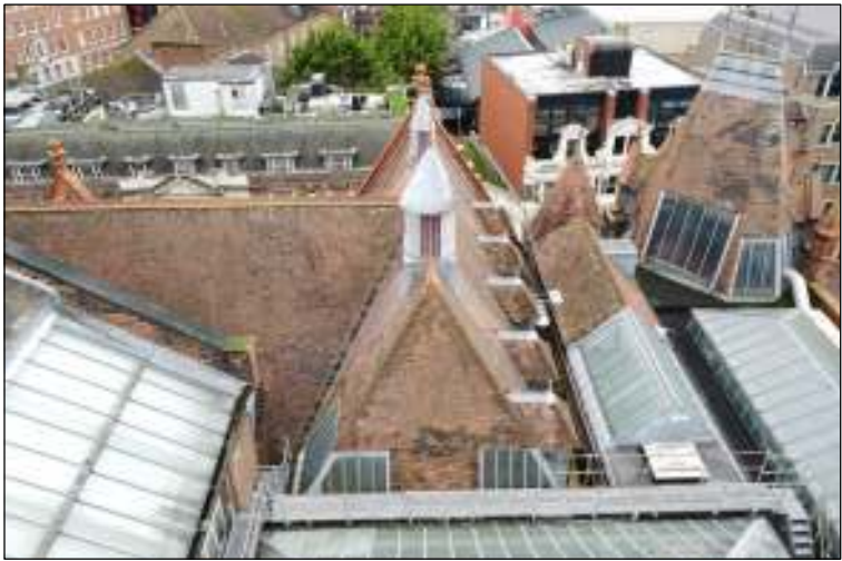
01 EAST HIPPED ROOF SLOPE RF7B NTS - Date Taken: 09/10/24
