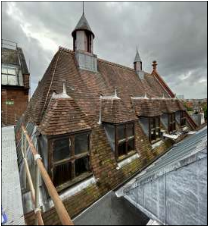
04 NORTH SLOPE RF7A AND DORMERS NTS - Date Taken: 08/10/24
