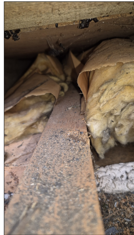
06 INSULATION BETWEEN RAFTERS NTS
