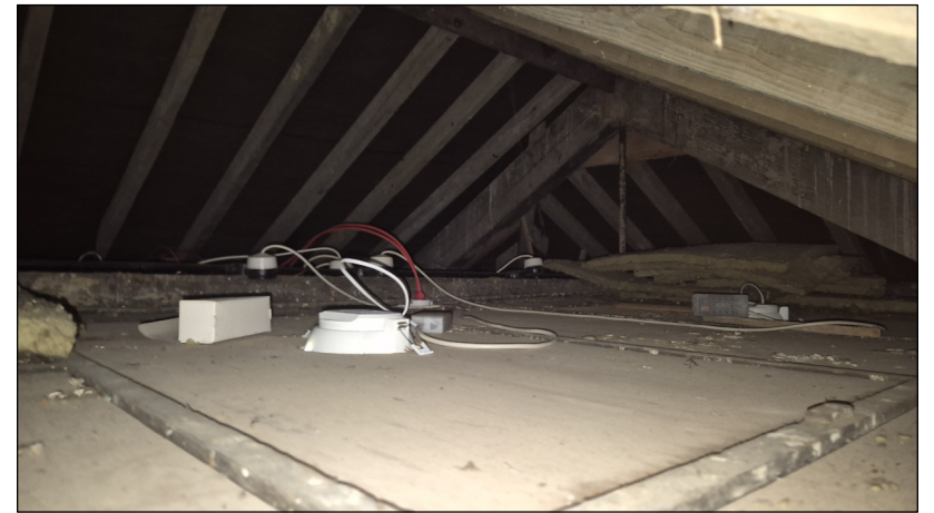
07 UNINSULATED ROOF VOID NTS
