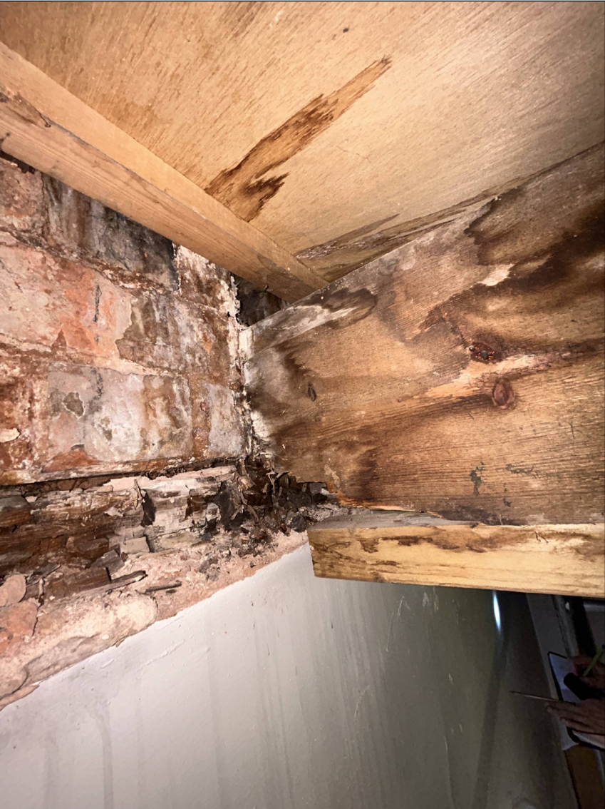
07 ROTTEN TIMBER JOIST AND WALL PLATE
