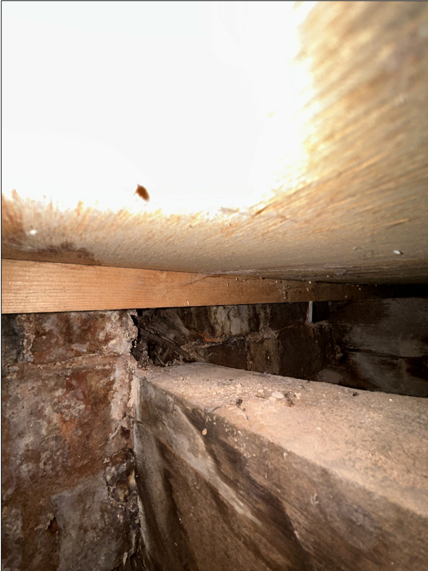
08 TOP OF DROPPED ROTTEN TIMBER JOIST
