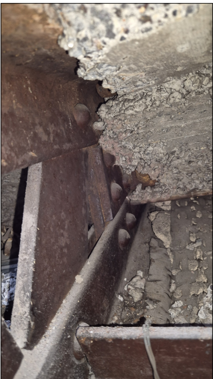
11 INVESTIGATION NO. 3 STEELWORK NTS
