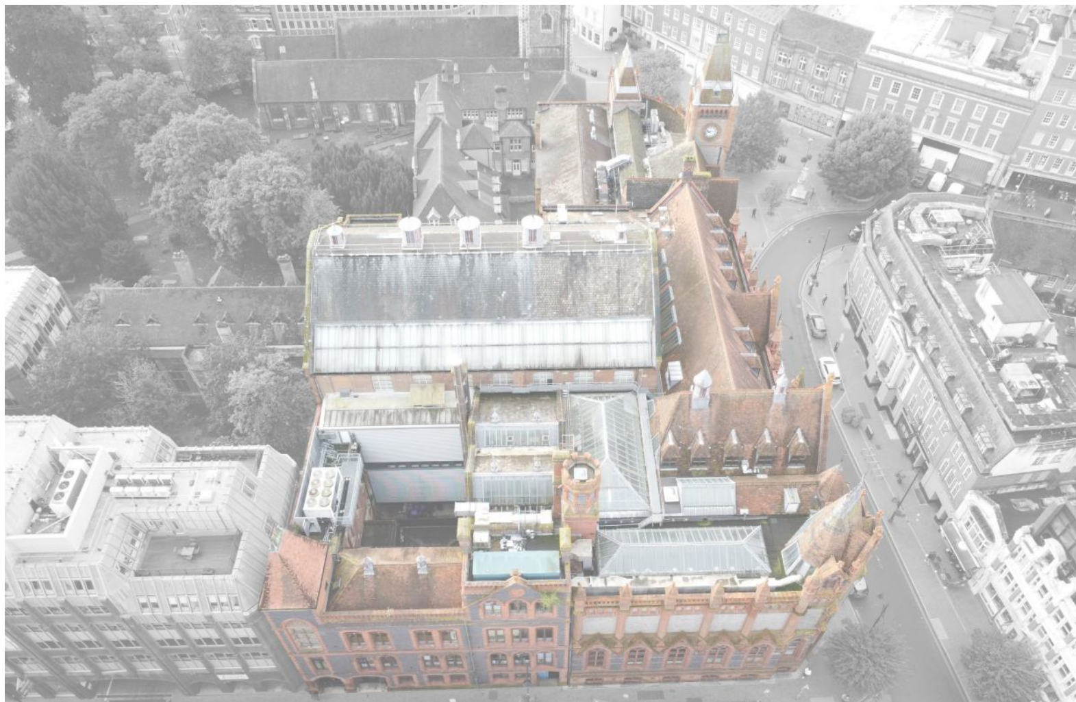
AERIAL VIEW OF TOWN HALL ROOFS. ROOF OVER THE MUSUEM IN THE FOREGROUND
