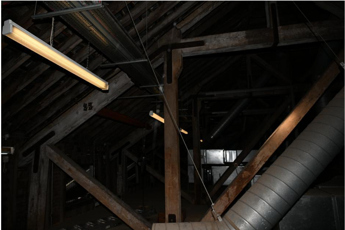
Image 13 Internal structure over concert hall
