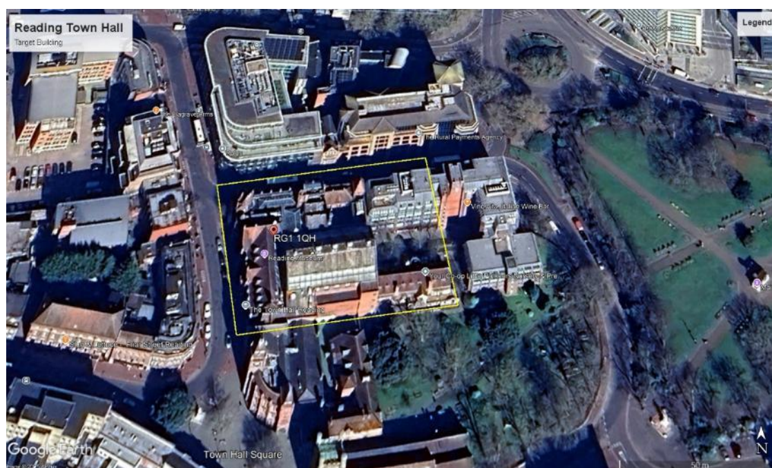
FIGURE 1. Target Building indicated by the yellow line above.
