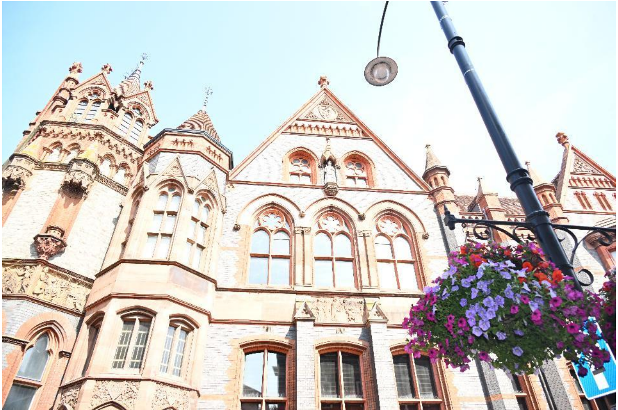
Image 3 Target Building roof structures
