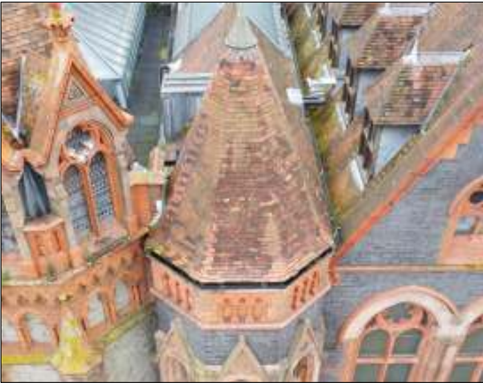
03 WESTERN ROOF SLOPES RF9 NTS - Date Taken: 09/10/24
