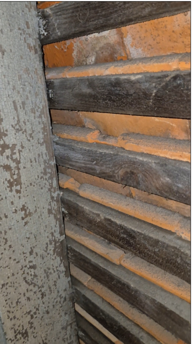
08 ROOF COVERING AND RAFTER
