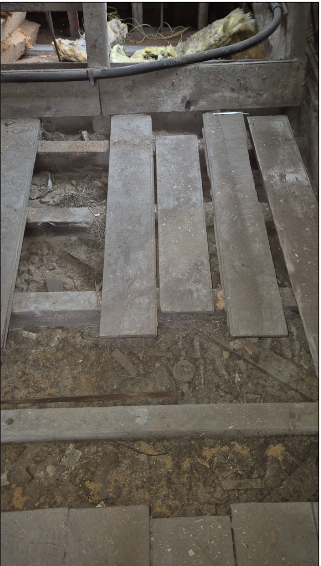
07 FLOOR JOISTS AND BOARDS
