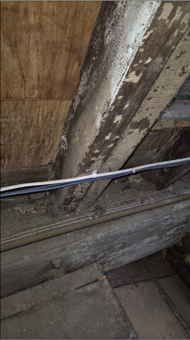
05 TIMBER RAFTERS DOUBLED UP AROUND PATENT GLAZING
