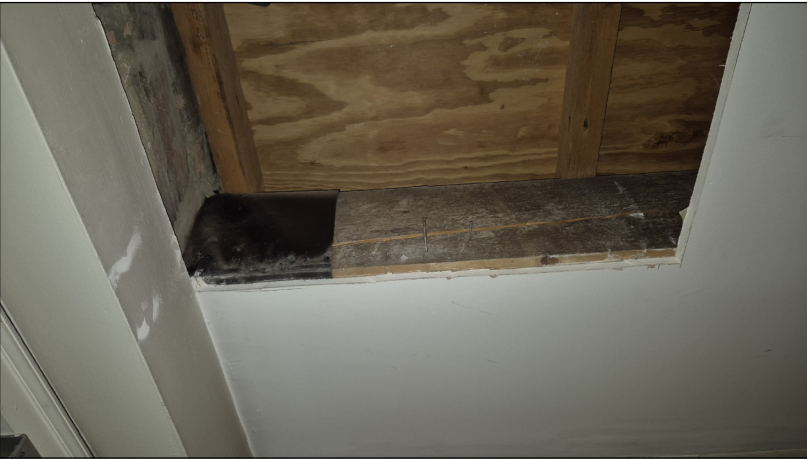
07 EXISTING FLAT ROOF JOISTS NTS
