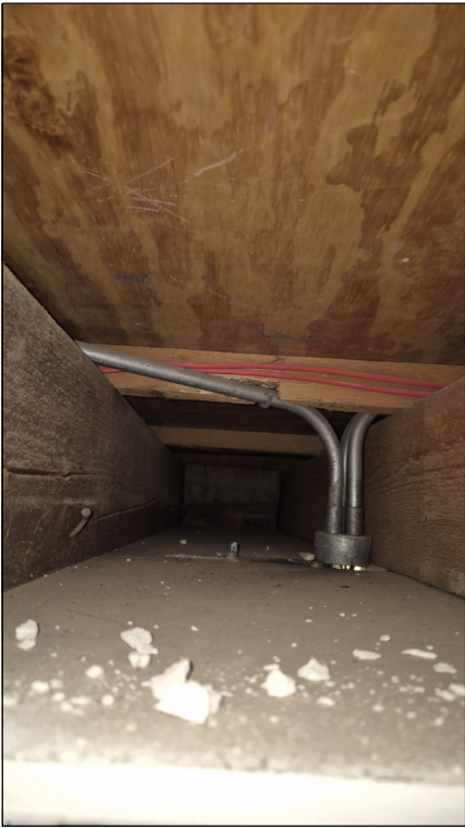
05 UNINSULATED ROOF VOID NTS
