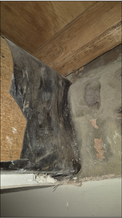
06 DAMP PROOFING TO TIMBER JOISTS NTS
