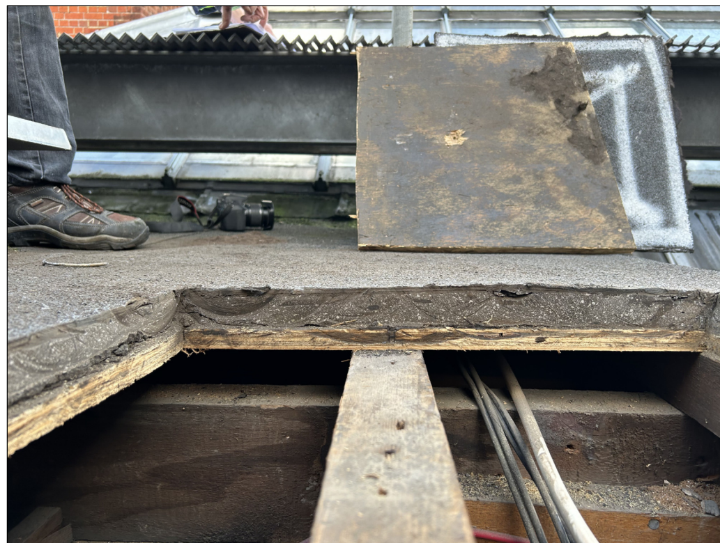
07 EXISTING FLAT ROOF COVERING MATERIALS NTS
