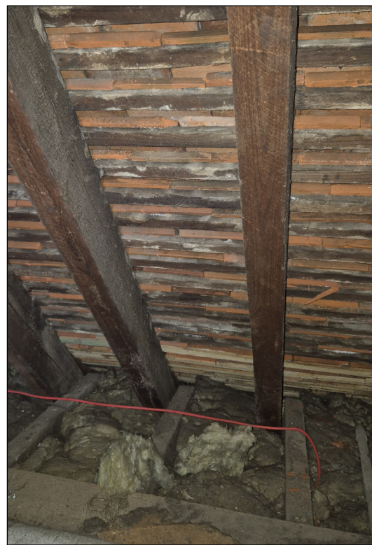
09 EXISTING TILED ROOF NTS
