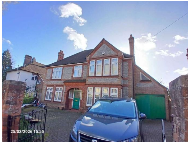
Photo 1: B1 - eastern elevation
