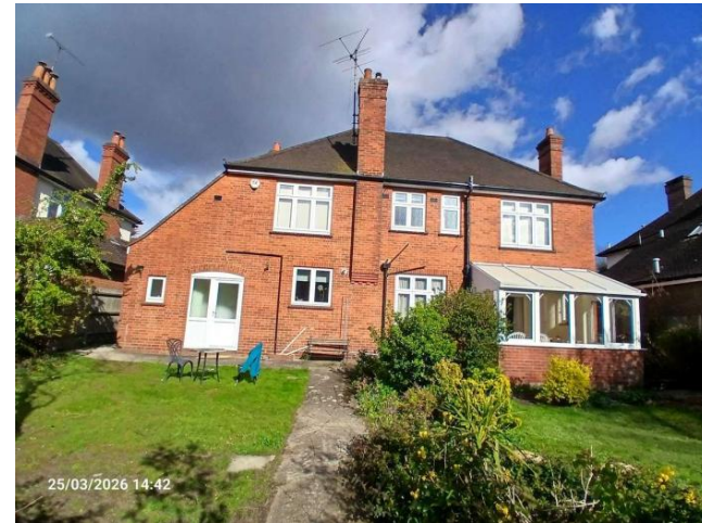
Photo 2: B1 - western elevation
