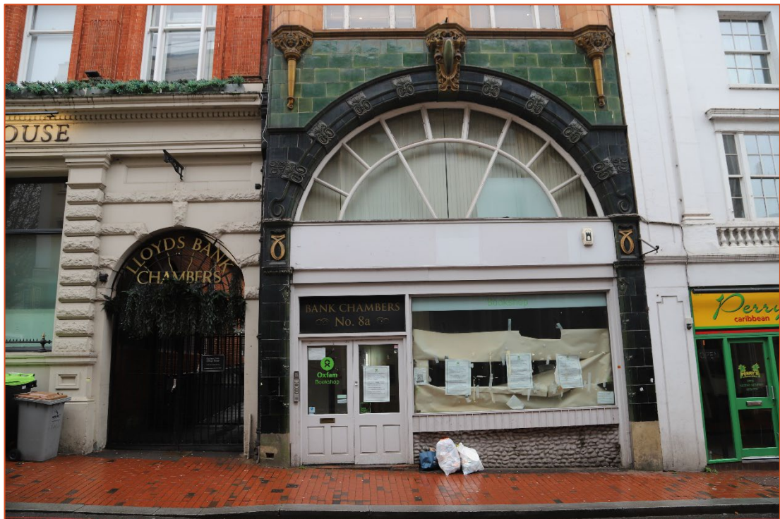
Plate 1 Looking east towards 8 High Street, 7 High Street and 1-2 Market Place (24mm)
