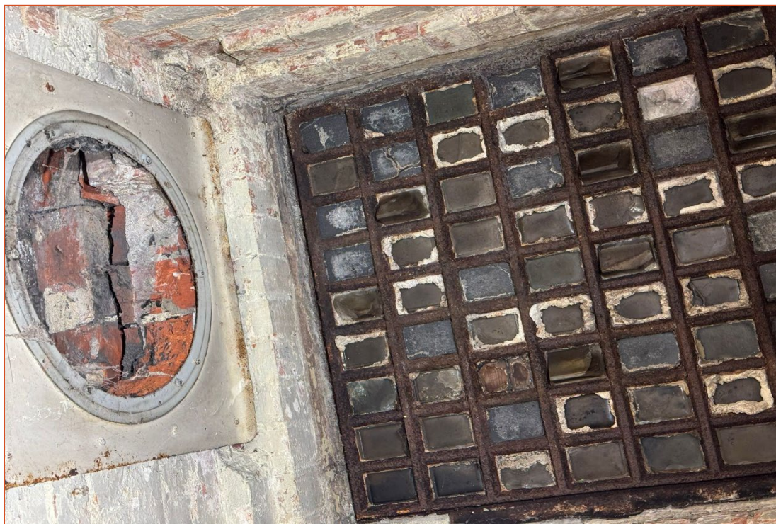
Plate 8 View of glass filled metal grate from basement and circular vent (24mm)
