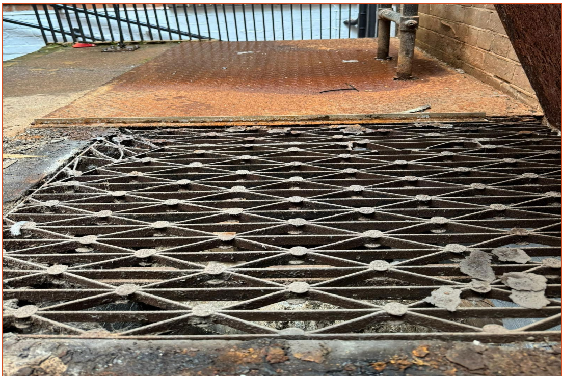
Plate 7 View of metal grate in courtyard (24mm)
