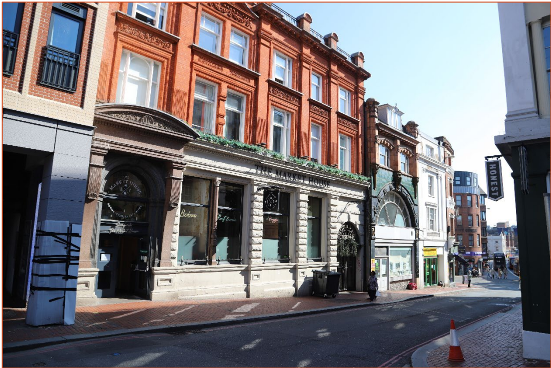
Plate 12 Looking south east towards 1-2 Market Place, and 7 and 8 High Street (24mm)
