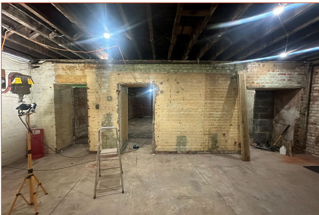
Plate 9 Looking west through the basement (24mm)
