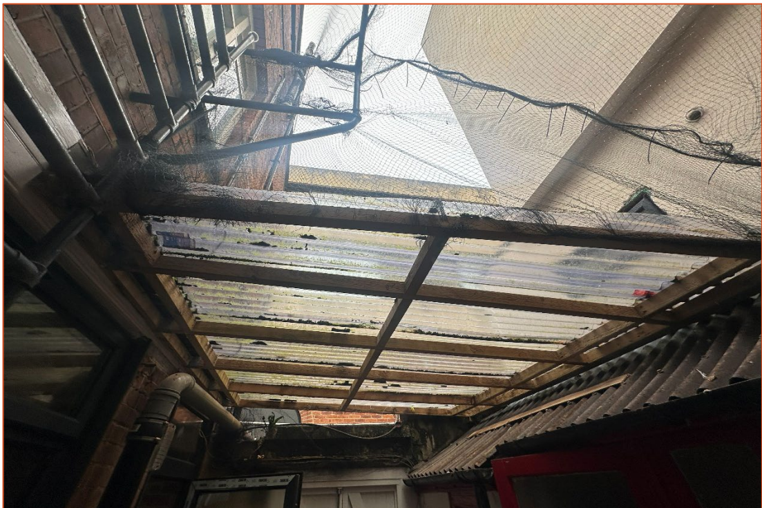
Plate 5 View of the modern leanto to the rear of the building (24mm)
