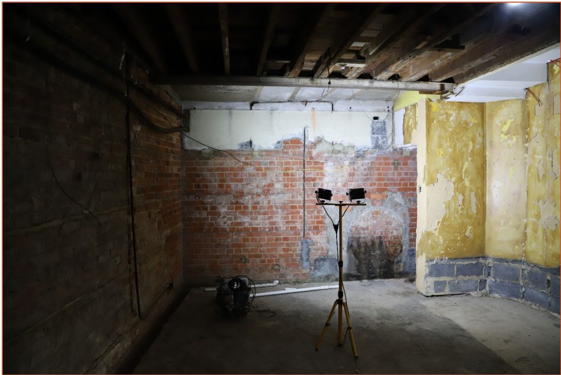
Plate 10 Looking west through the basement (24mm)
