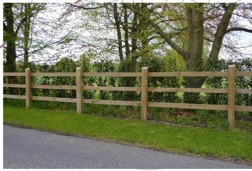
1.1m high softwood post and rail fencing
