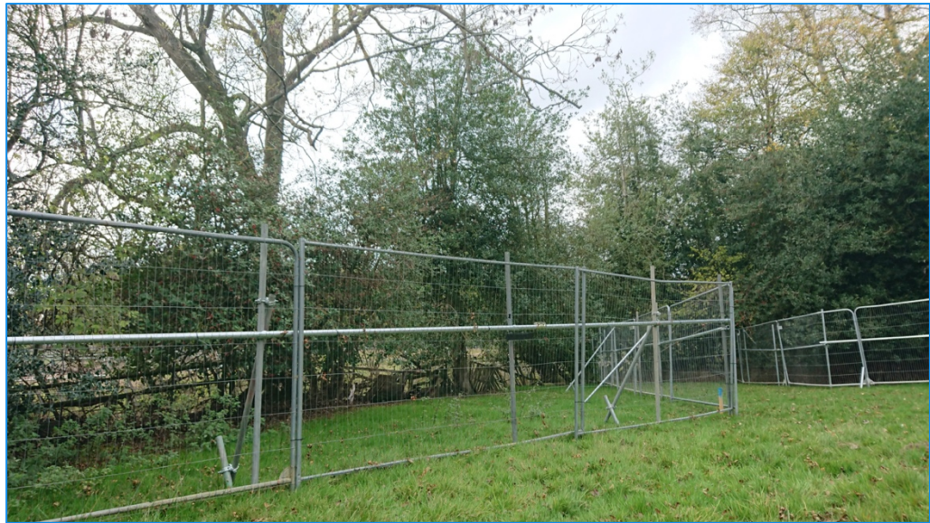
Typical tree protection barrier construction
